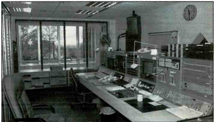
All programs are routed through master control to the proper transmitter site.
